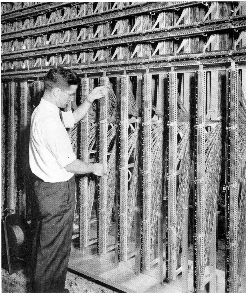
Assignment distribution frame for crossbar toll
