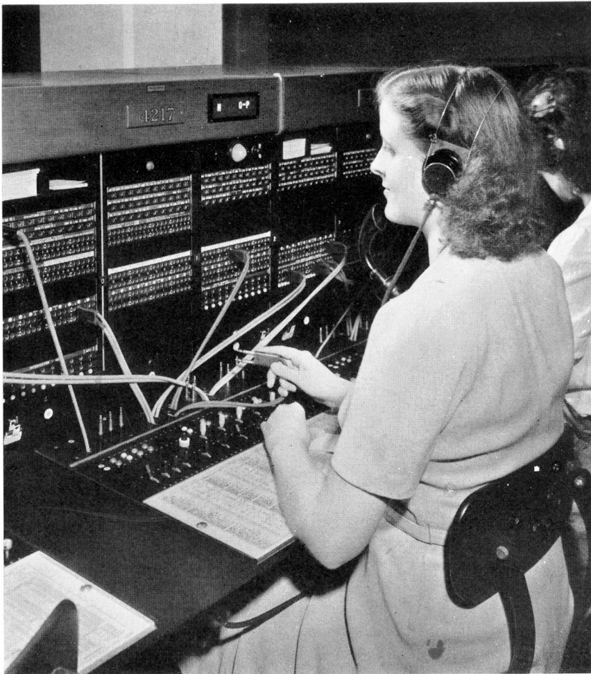
Fig. 3—The No. 5 toll switchboard for handling delayed calls
