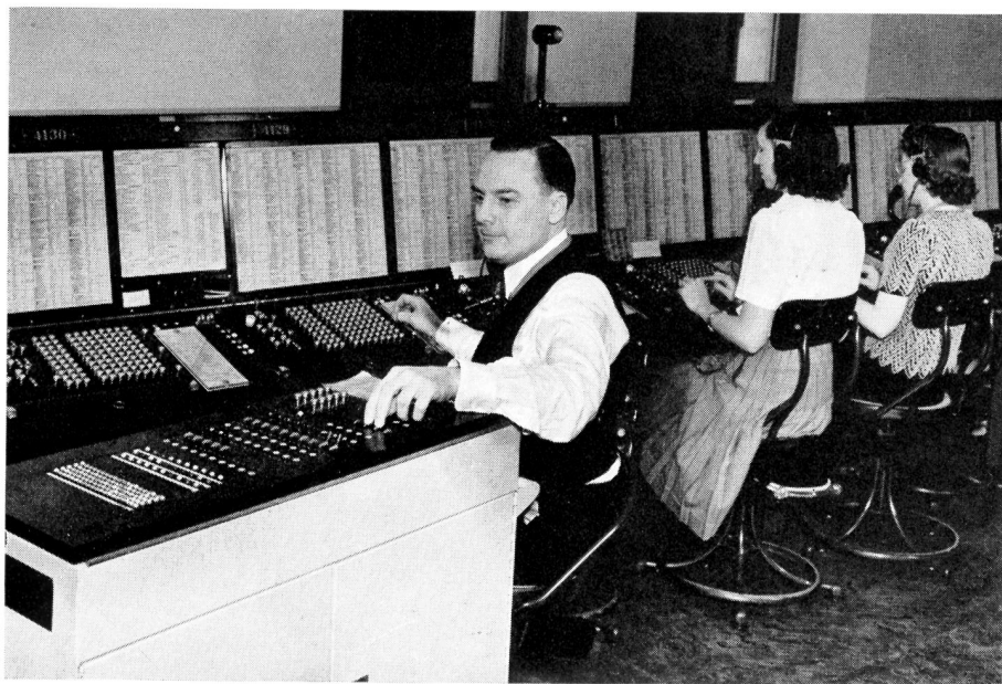
Test set for No. 4 switchboard positions
